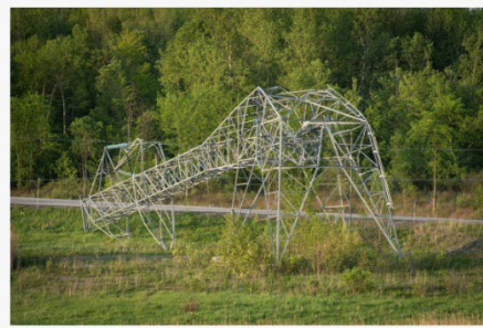
May 2022, derecho wind storm damages power lines and transmission tower
