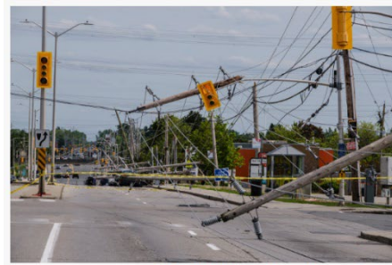
May 2022, derecho wind storm damages power lines and transmission tower
