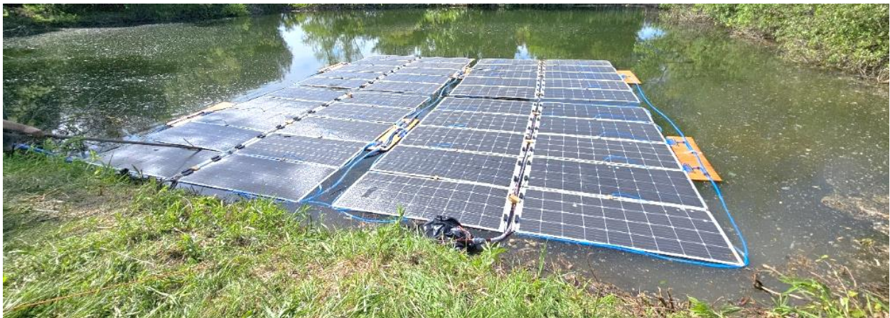
Figure 4.3.21 7kW FPV floating on the large pond at the ESW Field Station
