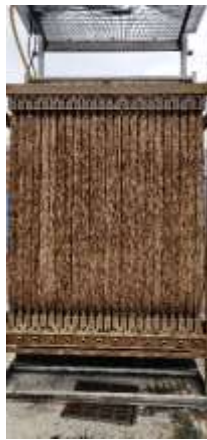
Figure 4: ZeeLung™ MABR Cassette After it has Been in Use (Tank 2 Cassette 6 Back, in cassette lifting on Nov 16, 2023 folder)
