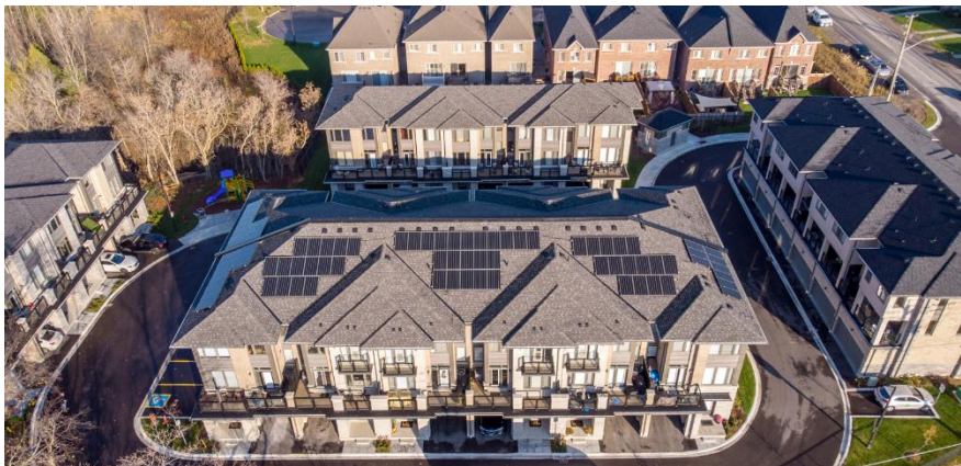
Aerial view of the completed Altona Towns development in Pickering, Ontario.
