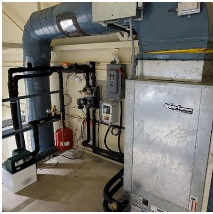
Figure 4: Newly installed variable speed geothermal heat pump
