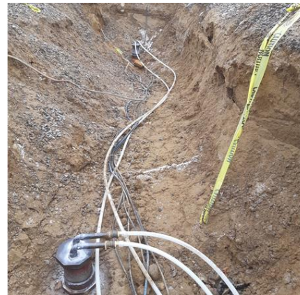
Figure 3: Supply and return lines connected to steel piles
