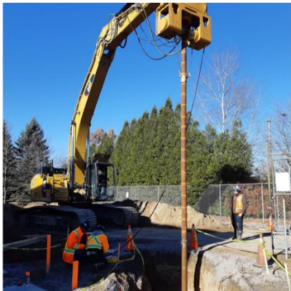
Figure 2: Installation of steel pile
