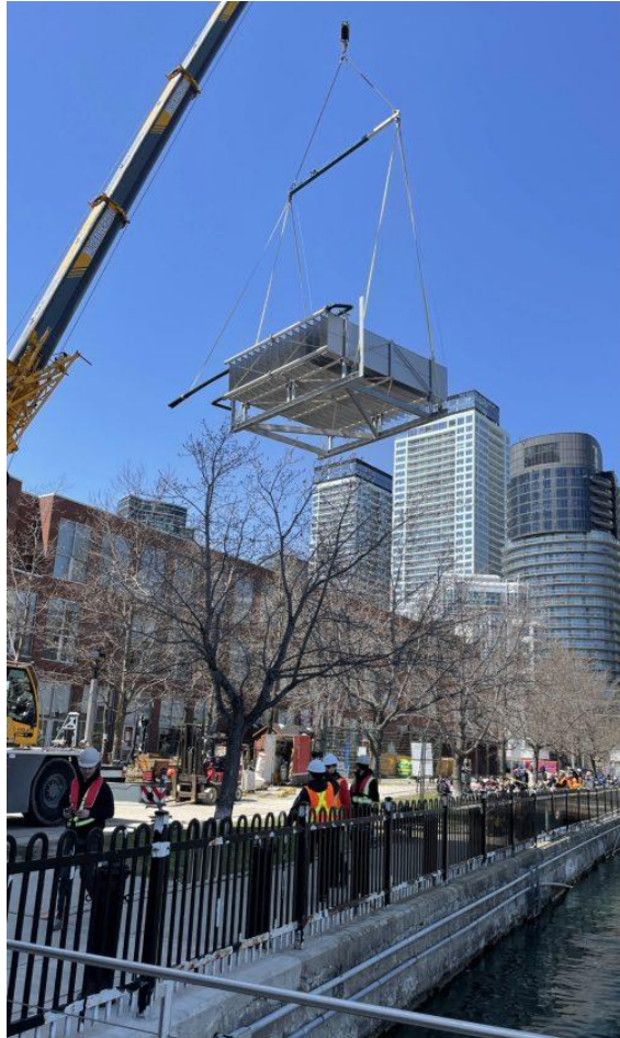
Cranes hoisting heat exchangers into Lake Ontario
