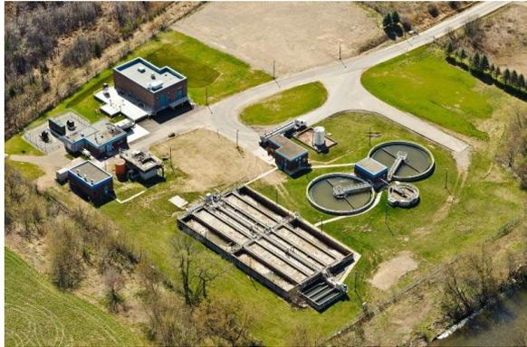
**Region of Waterloo:** The Region of Waterloo is replacing the aeration equipment at the Hespeler Wastewater Treatment Plant in Cambridge with Membrane-Aerated Biofilm Reactor (MABR) technology that is expected to reduce electricity and demand consumption. The project will quantify the energy and demand savings and greenhouse gas reduction resulting from the MABR technology.
