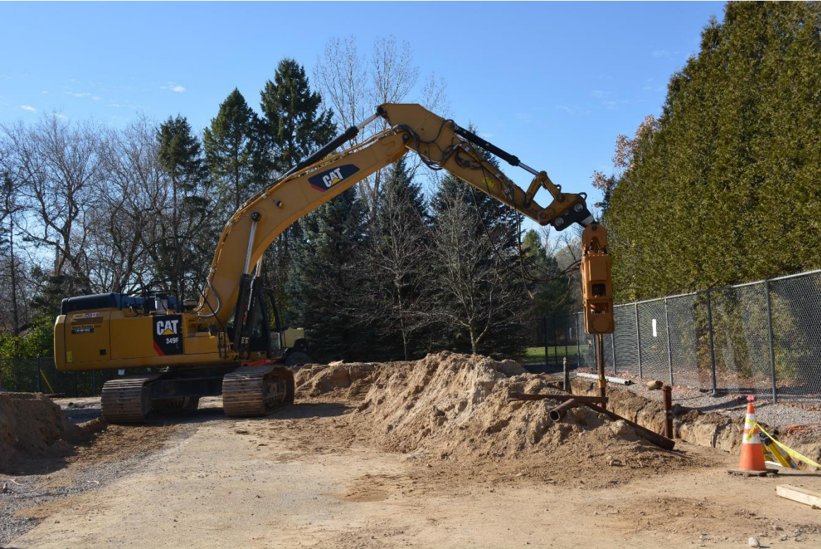
Installation of Innovia’s GEO system in Waterloo.
